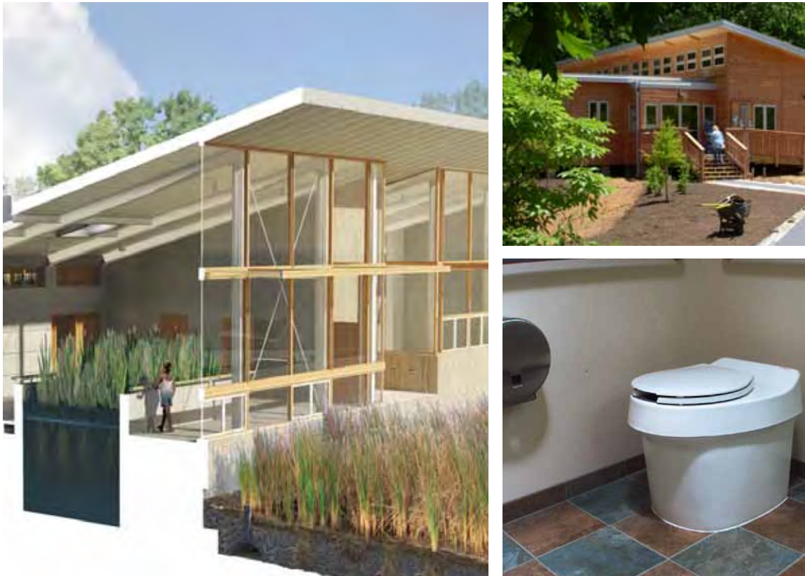
The first two certified Living Buildings in the United States, The Omega Center for Sustainable Living in Rhinebeck, NY (above left) and Tyson Research Center's Living Learning Center in Eureka, MO (above right) utilize different strategies to manage water and waste on-site. The Omega Center collects wastewater from the surrounding campus and treats it on-site through an eco-machine and constructed wetlands. Tyson's potable water is provided by a chemical-free rainwater harvesting system. The project includes composting toilets and a sub-surface constructed wetland to treat greywater. Images courtesy of BNIM Architects and Clivus Multrum.
