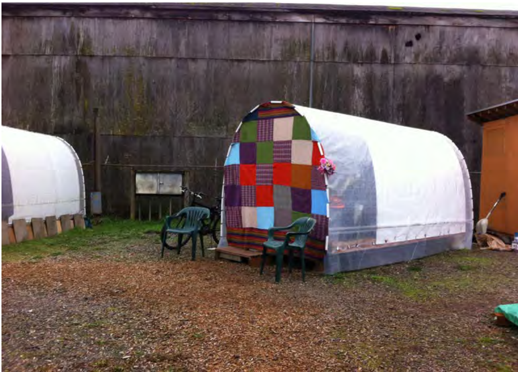
Opportunity Village in Eugene, Oregon. These conestoga-inspired tiny homes are made from a metal frame and plastic sheeting.
