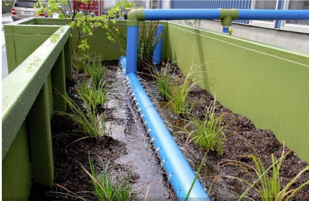
Gravity Feed from Roof Downspouts and Pumping from Oil/Water Separator
