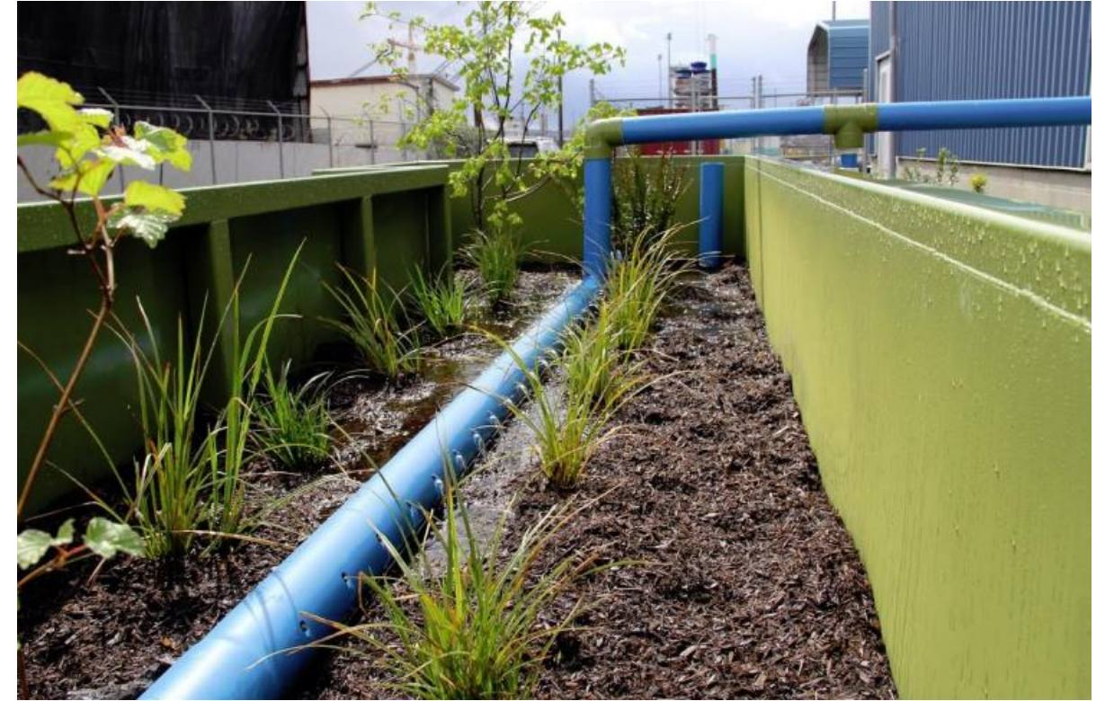
Gravity Feed from Roof Downspouts and Pumping from Oil/Water Separator
