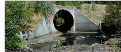
US 97 culvert that blocked fish passage at Butler Creek, a tributary to the Little Klickitat River near Goldendale.
