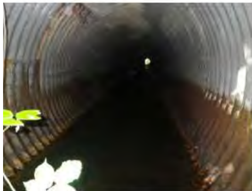
FISHER CREEK CULVERT
