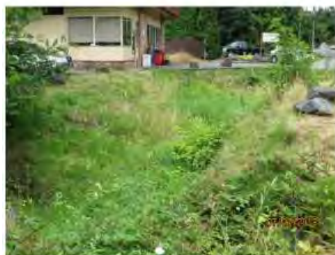
SR 104 LYON CREEK OUTLET
