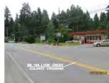
SR 104 LYON CREEK CULVERT CROSSING
