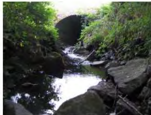
FISHER CREEK CULVERT OUTLET
