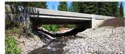
US 97 at Butler Creek after the $3.5 million barrier removal project was completed in April 2013.
