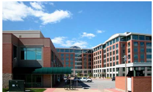
The TDS Business Center is located in a General Commercial District and includes some retail uses.
