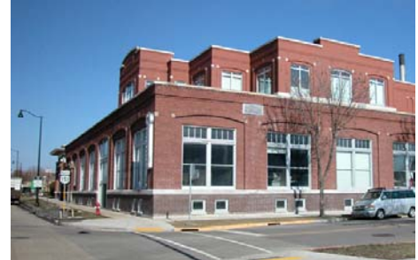
700 E. Washington Avenue has been adapted into a restaurant and entertainment space.
