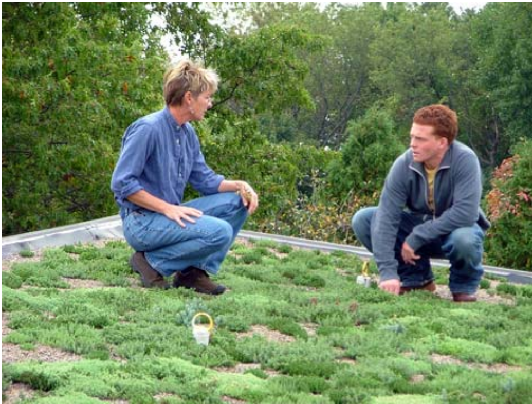
Green roofs are used to help reduce stormwater run-off and reduce heating and cooling costs for buildings.
