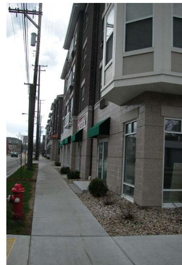
Student Apartments on Old University Avenue
