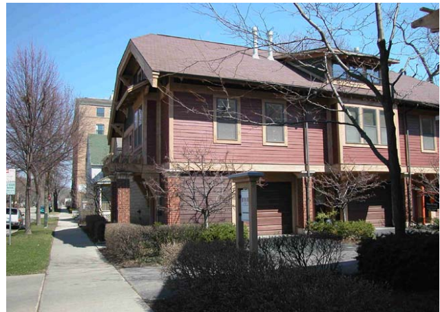
These townhouses were an infill project in the Tenney Lapham Neighborhood.
