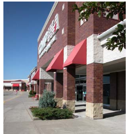
This retail strip center on Junction Road is in a General Commercial District.
