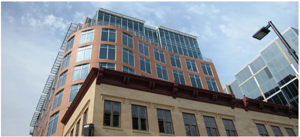
Block 89 Office Development
