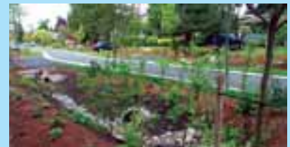
SeaStreet swale cleans and slows street runoff before it runs into Pipers Creek
