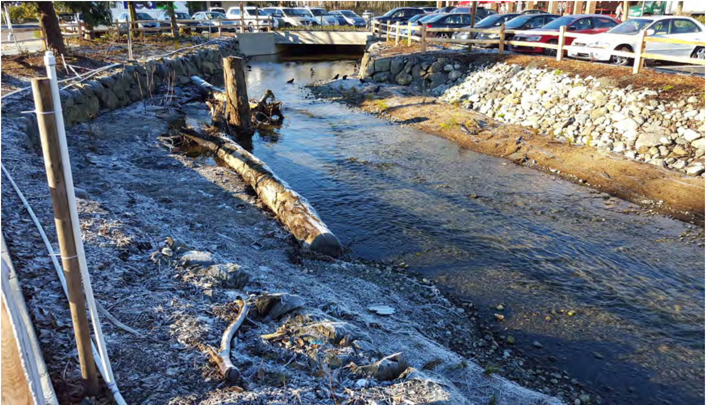
Completed Lyon Creek Flood Mitigation project
