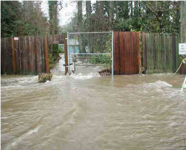
Culvert L40 (6-ft wide) – Private gate, flood event
