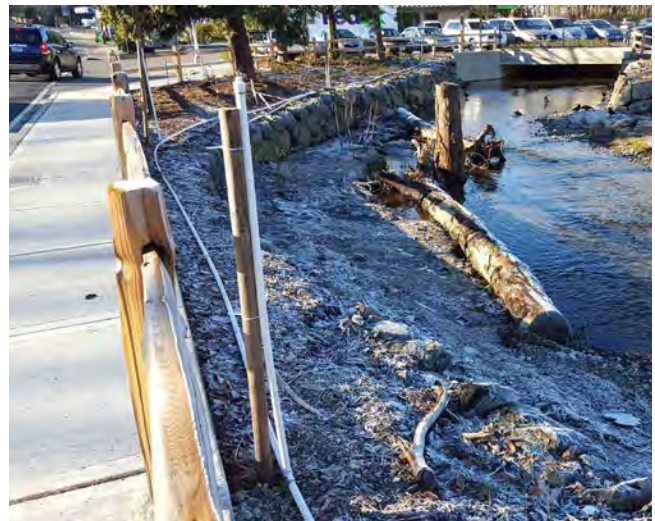
Culvert L30 (20-ft wide) -Channel widened, installation of woody debris and native plants; photo taken from new sidewalk on a winter day
