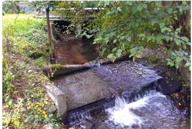
Fish barrier weirs removed by the project, downstream of culvert L10 (SR 522)
