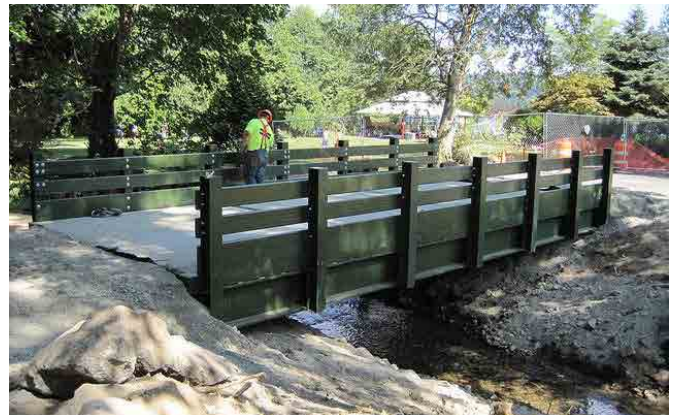
Phase II: Lake Forest Park Civic Club vehicle bridge installation
