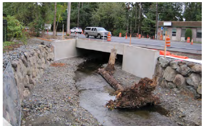
Phase IV: 40-ft open channel between culverts L10 and L20
