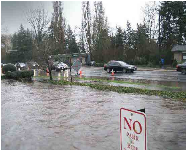
Upstream of culvert L20 (6-ft wide) – Flood event
