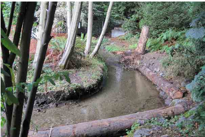
Phase I: Anchored woody debris armoring
