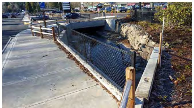
Sidewalk/viewing area adjacent to SR 522 after completion
