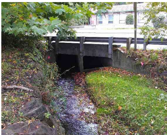
Culvert L10 (8-ft total width) – SR 522
