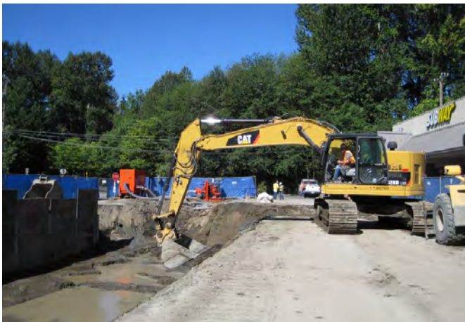
Phase V: Excavation for Culvert L30, 150-ft culvert length
