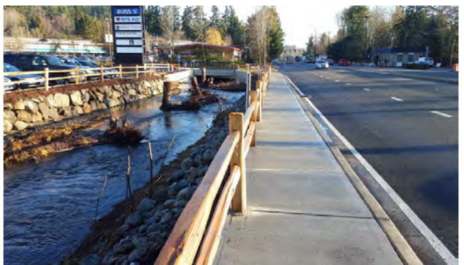
New sidewalk adjacent to SR 522 after project completion
