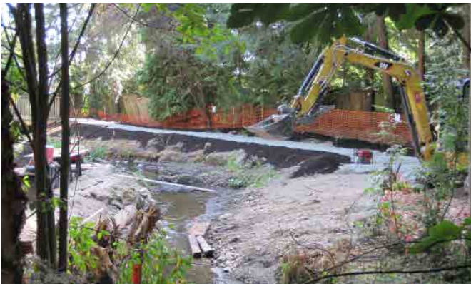
Phase I: Lyon Creek Waterfront Preserve stream armoring
