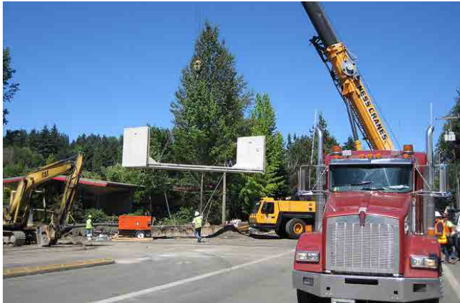
Phase III: L10 culvert sections placed during weekend highway closure
