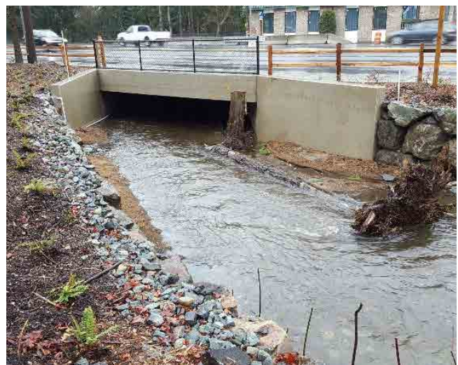
Culvert L10 (20-ft wide) – SR 522
