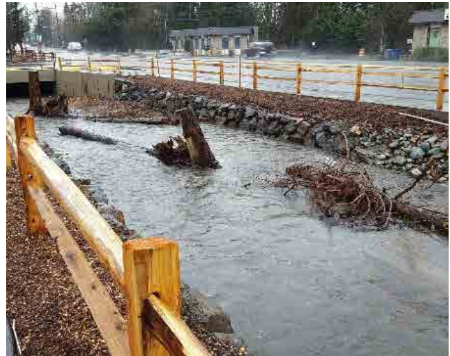
Culvert L20 (20-ft wide) - Channel widened, native plants and woody debris installed
