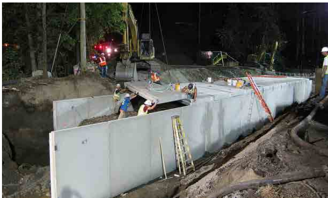
Phase III: SR 522 Culvert replacement, night work. Culvert replaced in 60 hours
