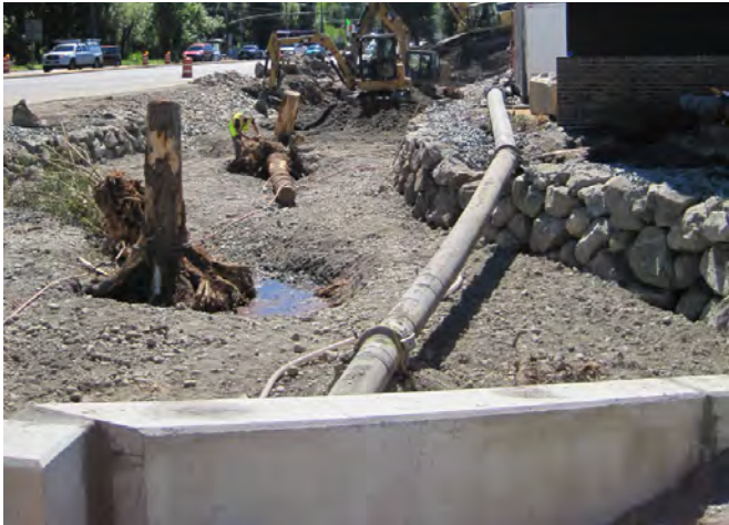
Phase V: 300-ft of open stream channel and setback retaining walls constructed, woody debris installed
