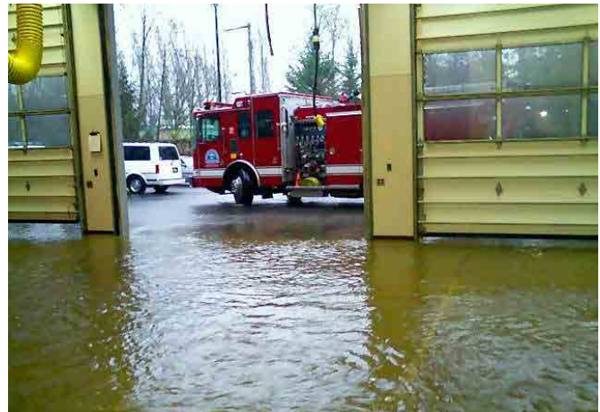
Flooded Northshore Fire Station, December 2007
