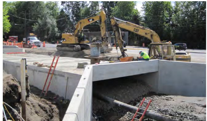
Phase IV: Culvert L20 installation and backfill
