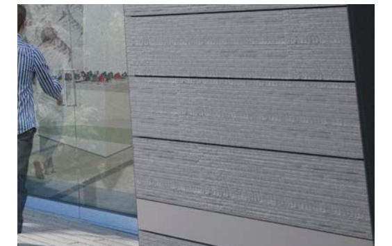
COMBED AND SMOOTH TERRA COTTA TILE WITH STEEL ANGEL FRAME
