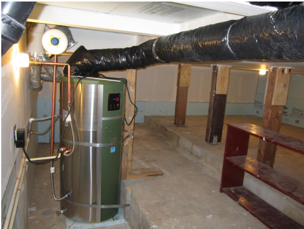
Heat Pump Hot Water Heater with duct bringing cold air to the exterior
