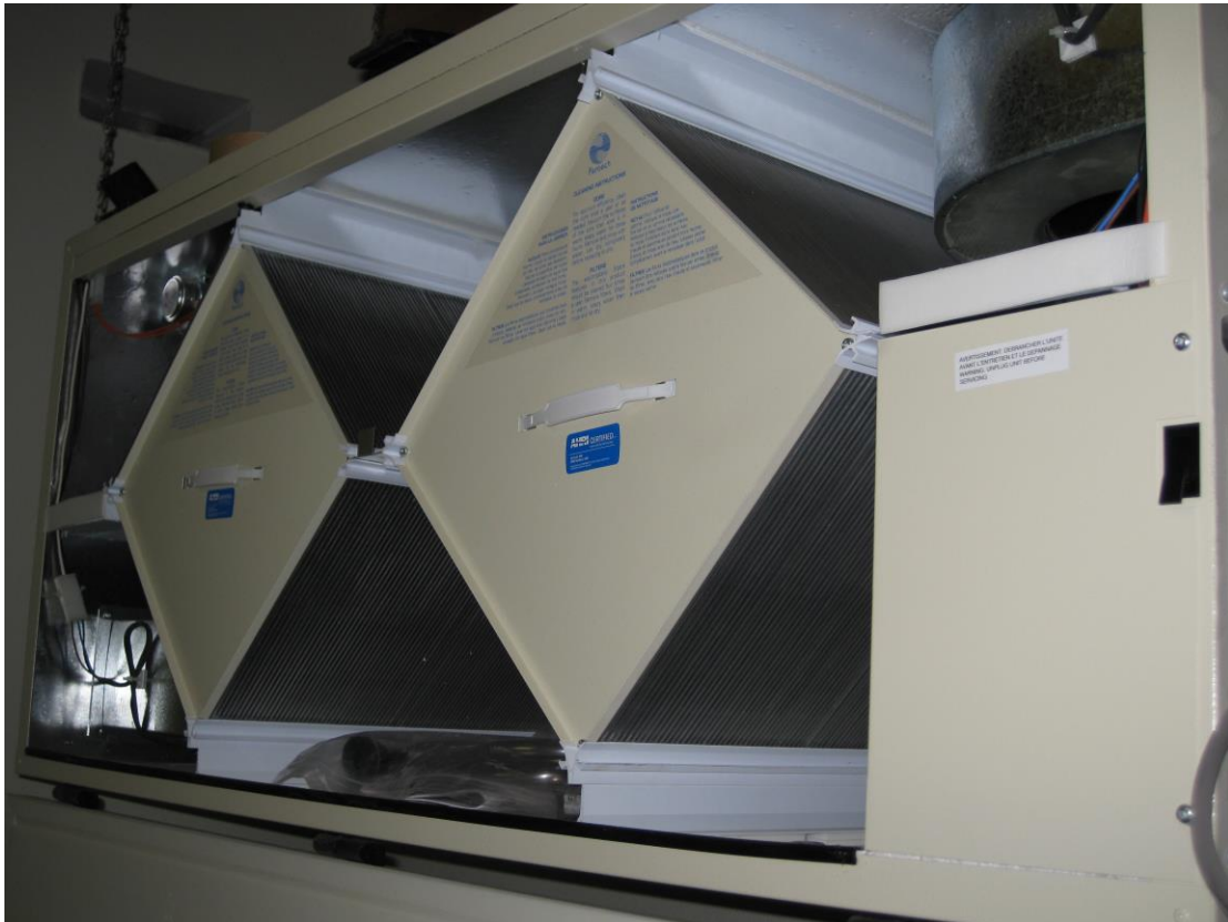
Inside the Fantech 3005R HRV with two heat exchange cores.
