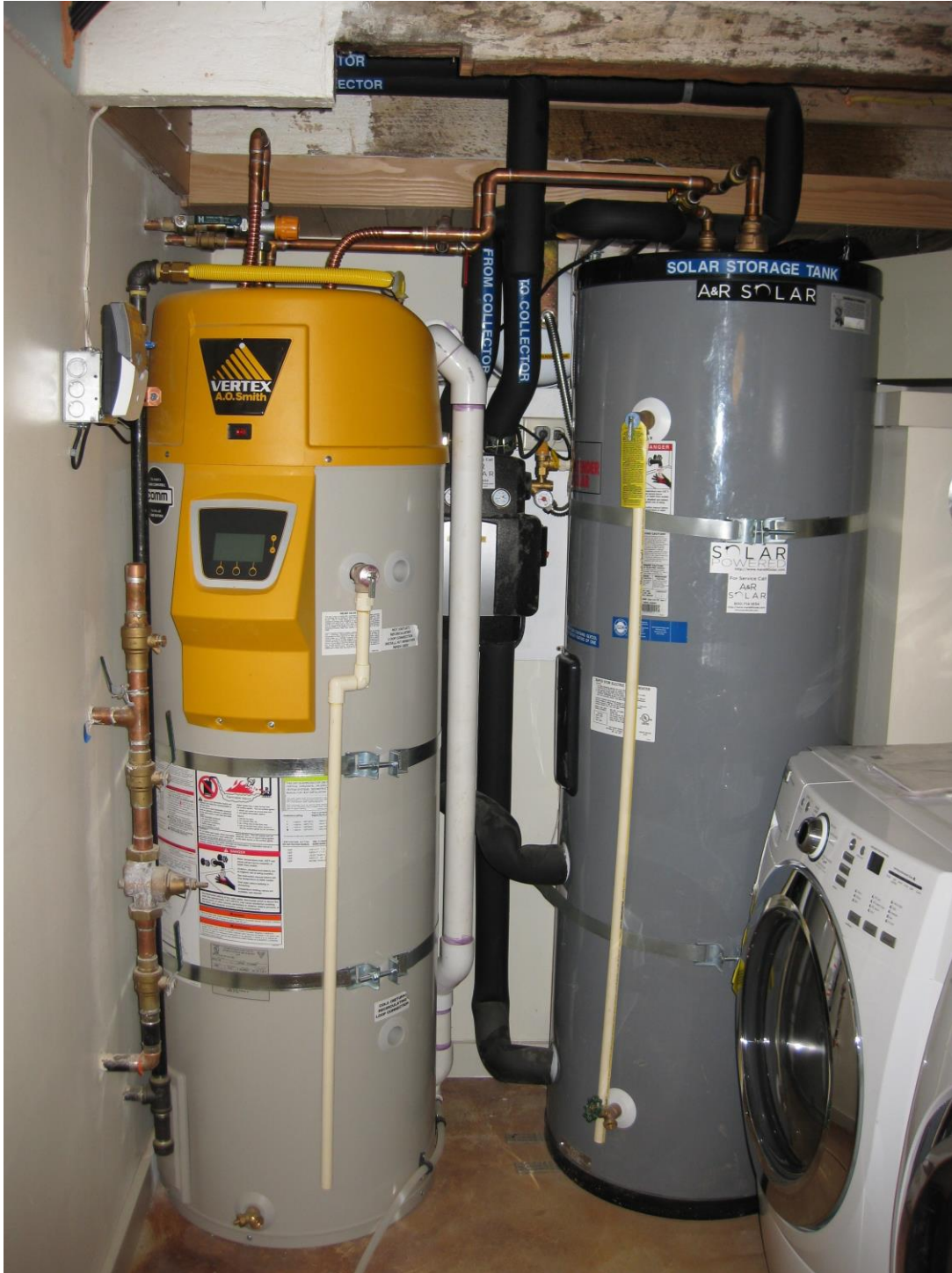
Solar Hot Water Storage paired with AO Smith Vertex Hot Water Tank
