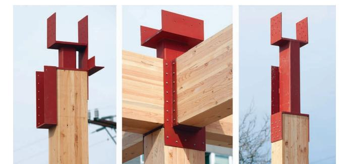
still have timber bearing on timber and the beams will not fail," said Court. "Each of the four beams passing through the bucket connection has about three inches of material bearing directly on the column below."
